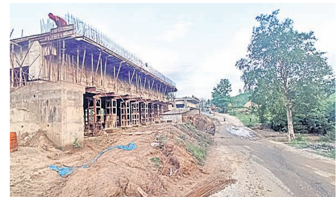
Construction of a bridge moving at a snail's pace in Kalimela
