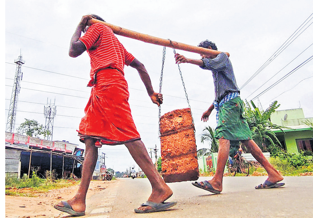
Two labourers carrying a block of stone across a road to a construction site in Angul town
