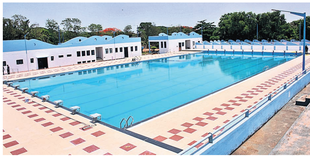
The newly-built swimming complex at the Kalinga Stadium is all set to welcome back the swimmers
