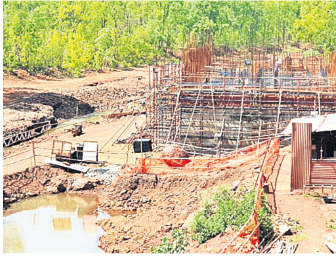
The under-construction dam across river Suna.
