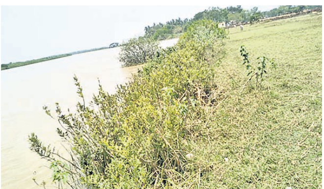
Unprotected banks of Salandi.
