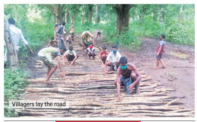
Villagers lay the road
