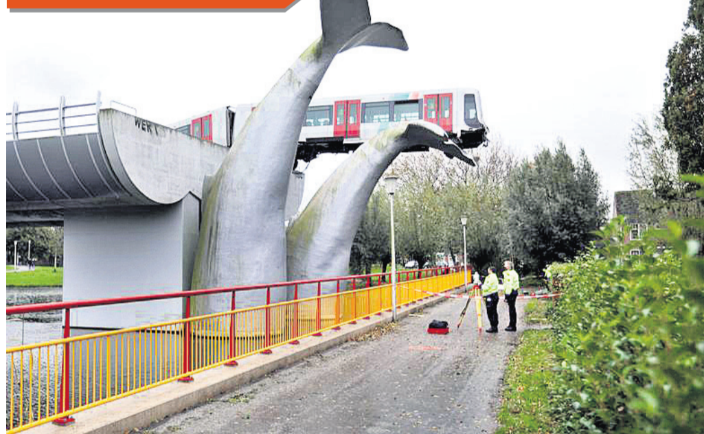
An elevated train that crashed through a stop block and landed on a whale tail sculpture at De Akkers subway station in Spijkenisse, near Rotterdam, Netherlands
