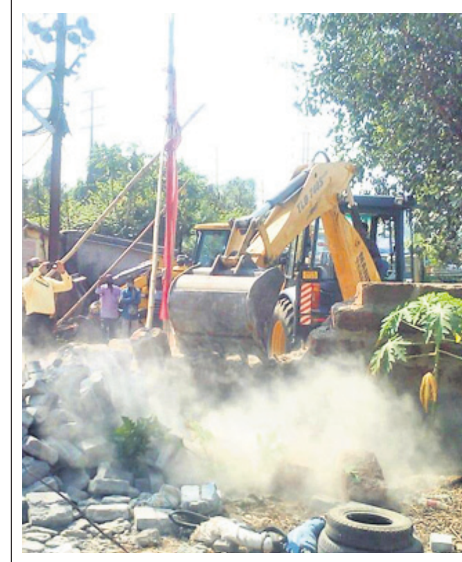
Civic officials demolish illegal structures at Aiginia in Bhubaneswar, Tuesday
