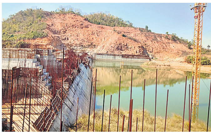
then start the dam work.
