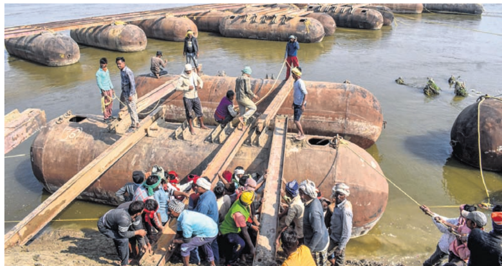
Labourers make a temporary pontoon tank bridge over Ganga river for the upcoming Magh Mela festival amid coronavirus pandemic at Sangam in Prayagraj, Saturday
