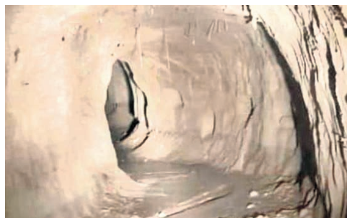
A view of the tunnel
