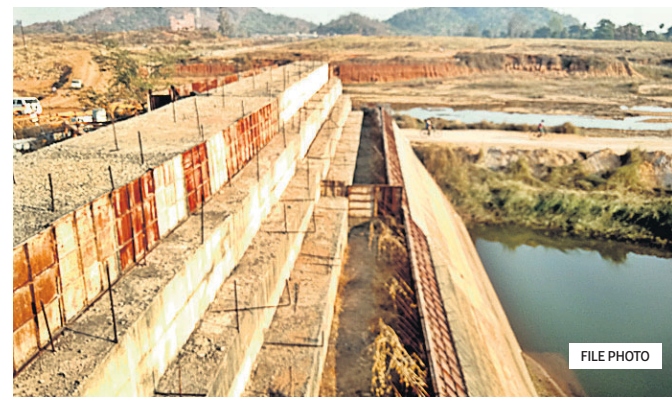
Lower Suktel Irrigation Project
