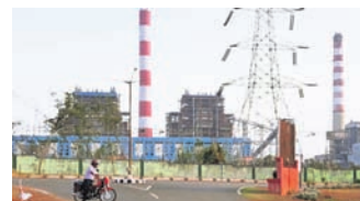
ceasing its unit in Angul district. Around 420 megawatt of power production was disrupted owing to disconnection of the OPGC unit alone, an official source said. On being informed about the dis-
