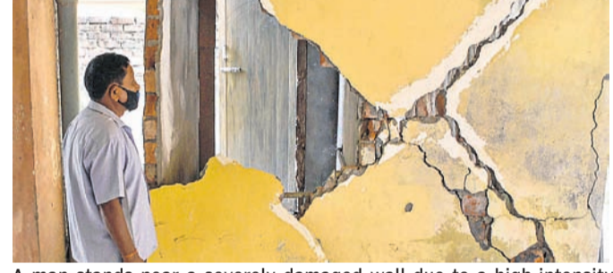
A man stands near a severely damaged wall due to a high-intensity earthquake, in Guwahati
