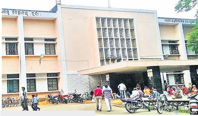
An oxygen refilling plant is already functional in Sambalpur while two others are in Jharsuguda. The three plants together can refill 2400 mega cylinders per day. They cater to the needs of patients in Sambalpur, Bargarh, Deogarh, Bolangir, Jharsuguda, Sonepur, Boudh and Nuapada
