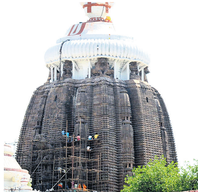
Repair work under way at Srimandir in Puri, Saturday
