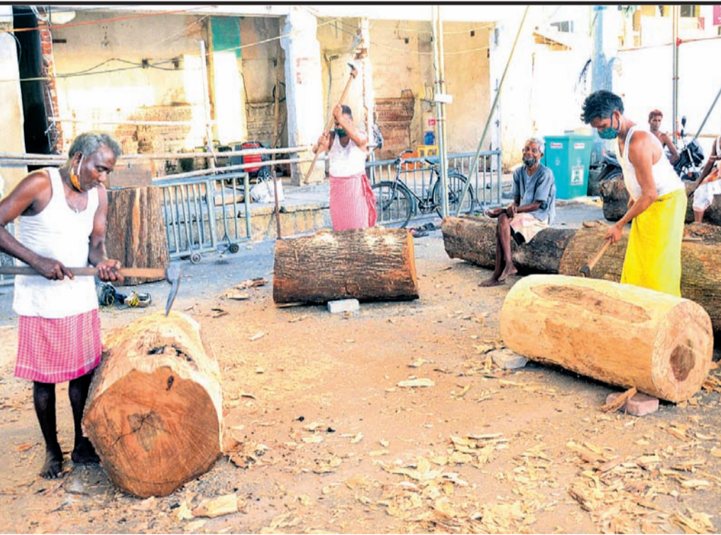
Carpenters shaping hubs as part of chariot construction work at Rath Yard in Puri, Tuesday
