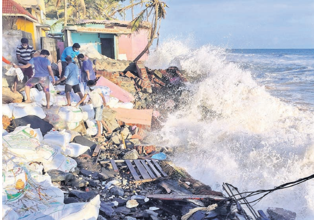
People place sand bags to create a temporary embankment along a beach during rough sea after damage to coastal areas by Cyclone Tauktae in Thiruvananthapuram, Tuesday.
