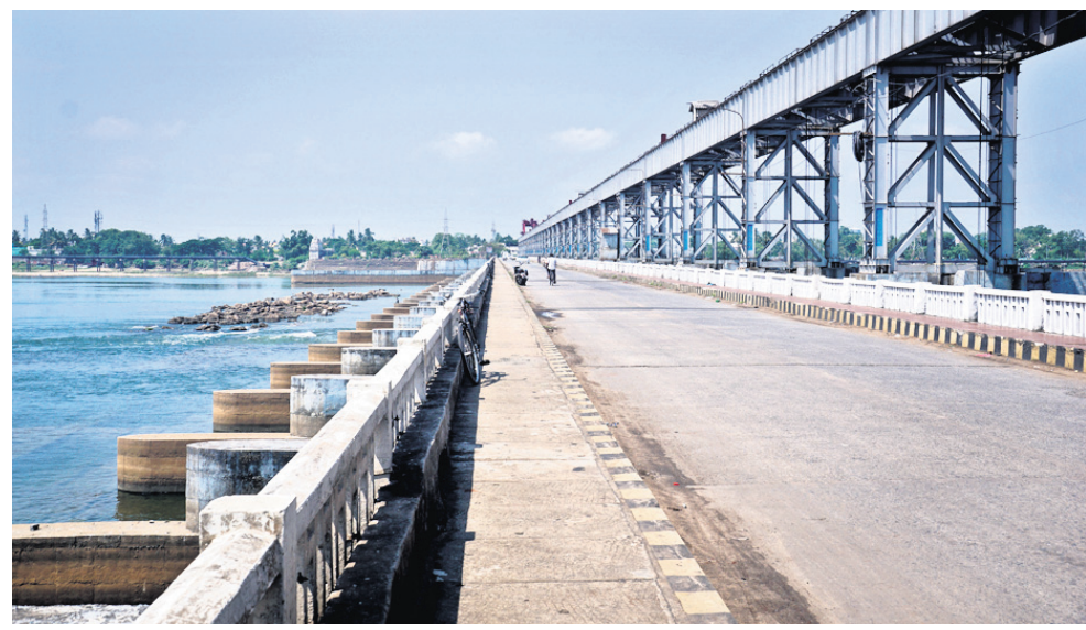
Rasulgarh overbridge in Bhubaneswar and Jobra anicut bridge in Cuttack (bottom) look empty as the urban areas of Odisha were put under weekend shutdown to tackle the second wave of Covid-19
