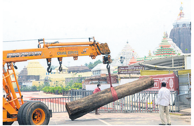
A crane being used to transport logs to Rath Yard
