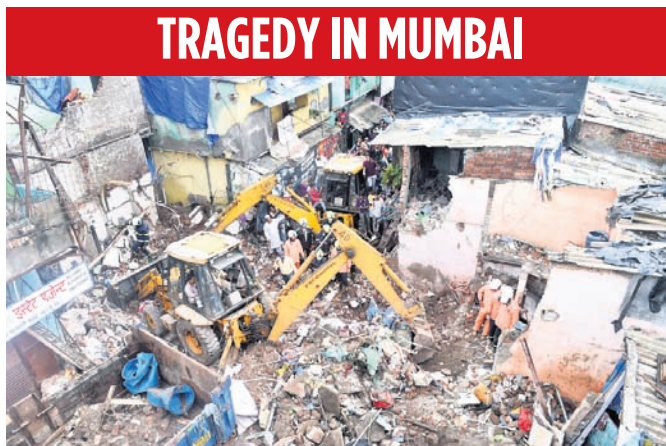
Rescue operation underway
