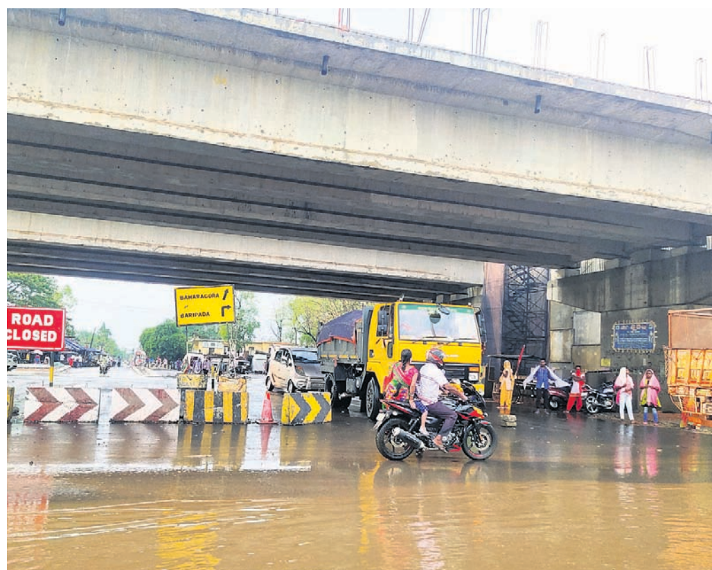
Motorists negotiating a flooded National Highway-49 at Bombay Square in Saraskana of Mayurbhanj district which was waterlogged due to lack of drainage facilities
