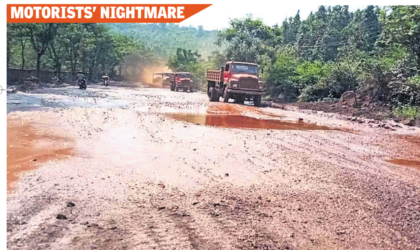
A stretch of Joda-Bamebari Express Road in Keonjhar district has turned into a death trap with no signs of improvement in road condition despite works going on for years
