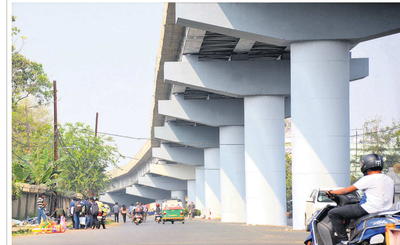
Even as the construction of a fly-over between Dhuchurapada Square and Kacheri Square in Sambalpur town has been completed, it is yet to be thrown open for public use
