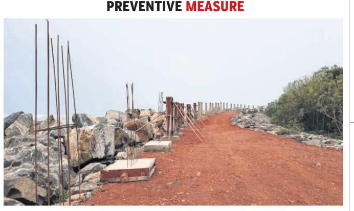
Construction of a wall underway on the stone embankment on Mahanadi river mouth near Nehru bungalow in Paradip to save the coastlines from erosion OP PHOTO
