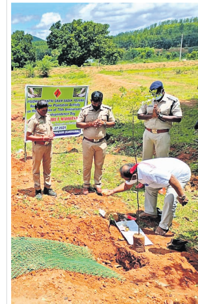
A plantation programme being launched alongside a PMGSY road in Khajuripada area in Kandhamal district
