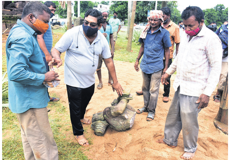
Civic authorities removing sculptures from Master Canteen Square in Bhubaneswar, Saturday, to pave way for the Smart Janpath project. A sculpture got broken during its relocation triggering sharp reactions from various quarters
