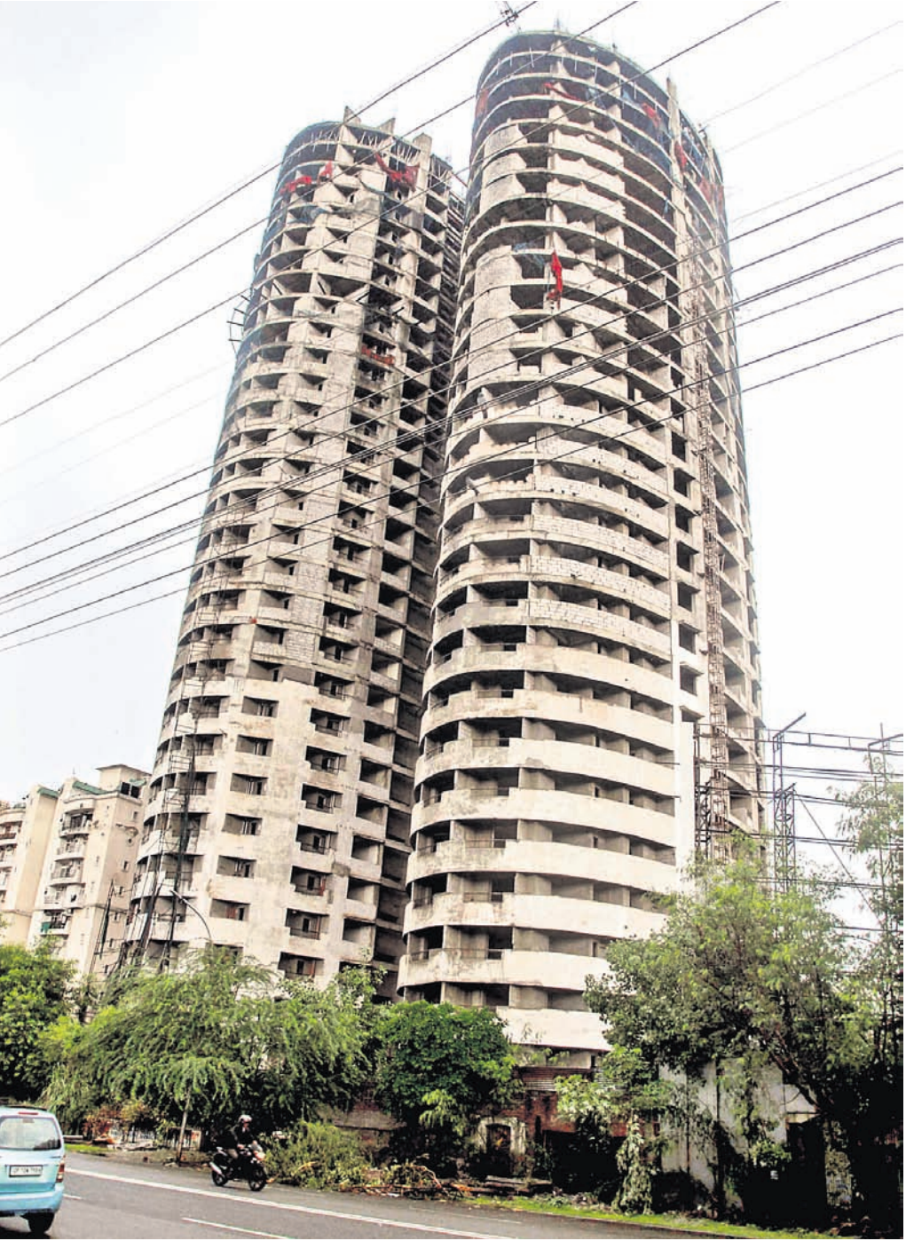
ILL-FATED A view of the 40-storey twin towers built by real estate company Supertech in Noida. The Supreme Court Tuesday directed demolition of the towers for violation of building by-laws
