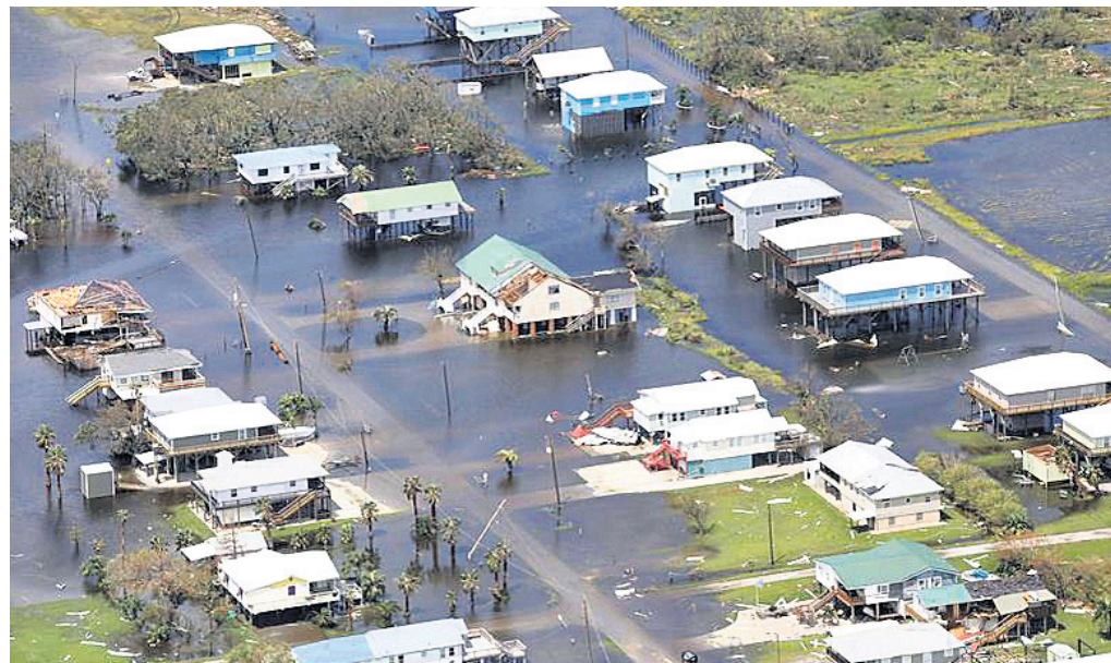
Ida leveled Grand Isle, a town of 740 on the edge of the Gulf of Mexico, where officials said virtually every structure sustained damage and about 40% were destroyed
