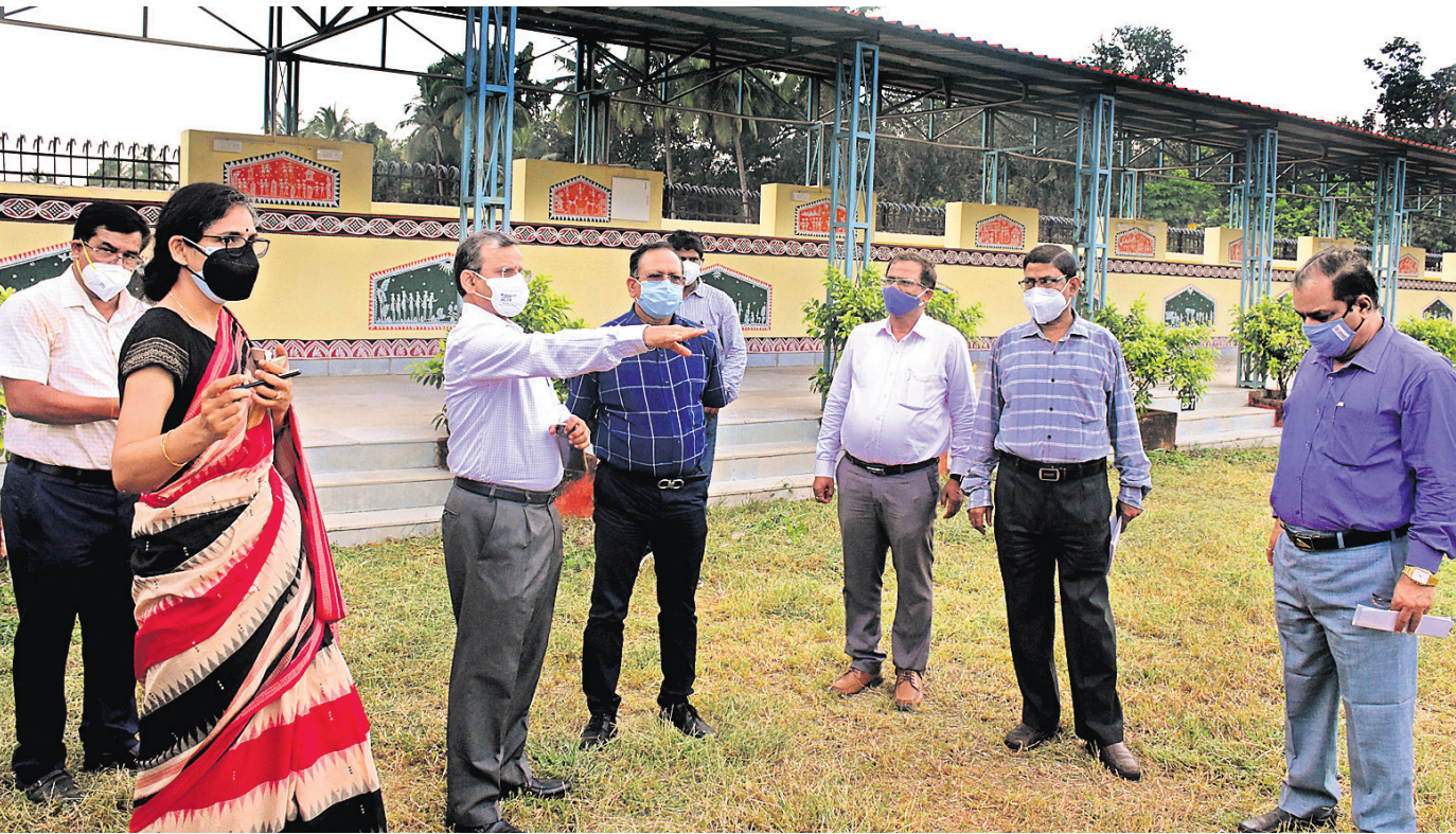
Chief Secretary Suresh Chandra Mahapatra along with Development Commissioner Pradeep Kumar Jena and Handlooms, Textiles and Handicrafts department Secretary Shubha Sharma inspecting the renovation work at Ekamra Haat in Bhubaneswar, Saturday
