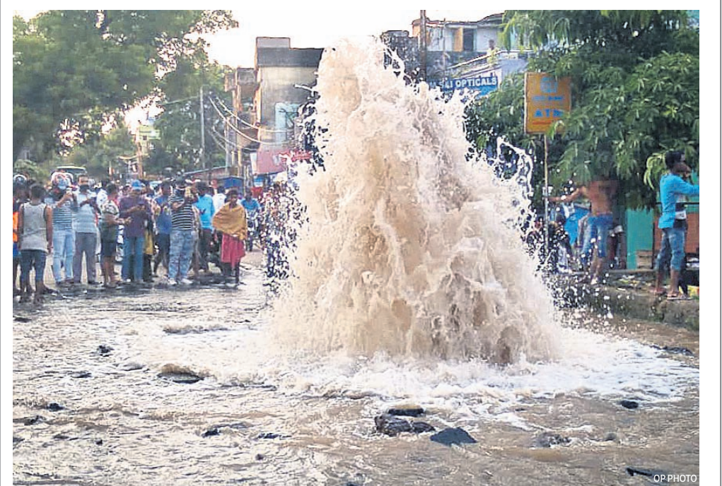
Water gushes out of a breach in the supply line underneath the Ring Road near Raja Bagicha in Cuttack, Wednesday
