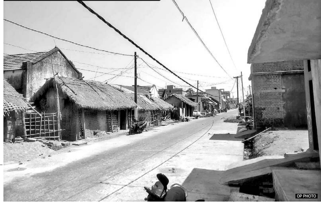
An overhead high transmission power cable hangs precariously on road posing serious threat to the lives of residents in Angapada village under Kishorenagar block in Angul district. The wire has been allegedly hanging for last one year
