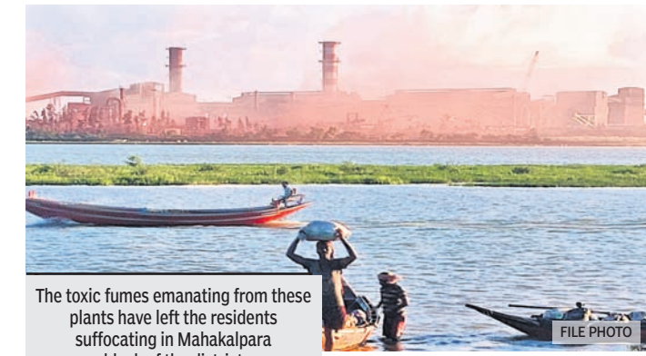
The toxic fumes emanating from these plants have left the residents suffocating in Mahakalpara block of the district
