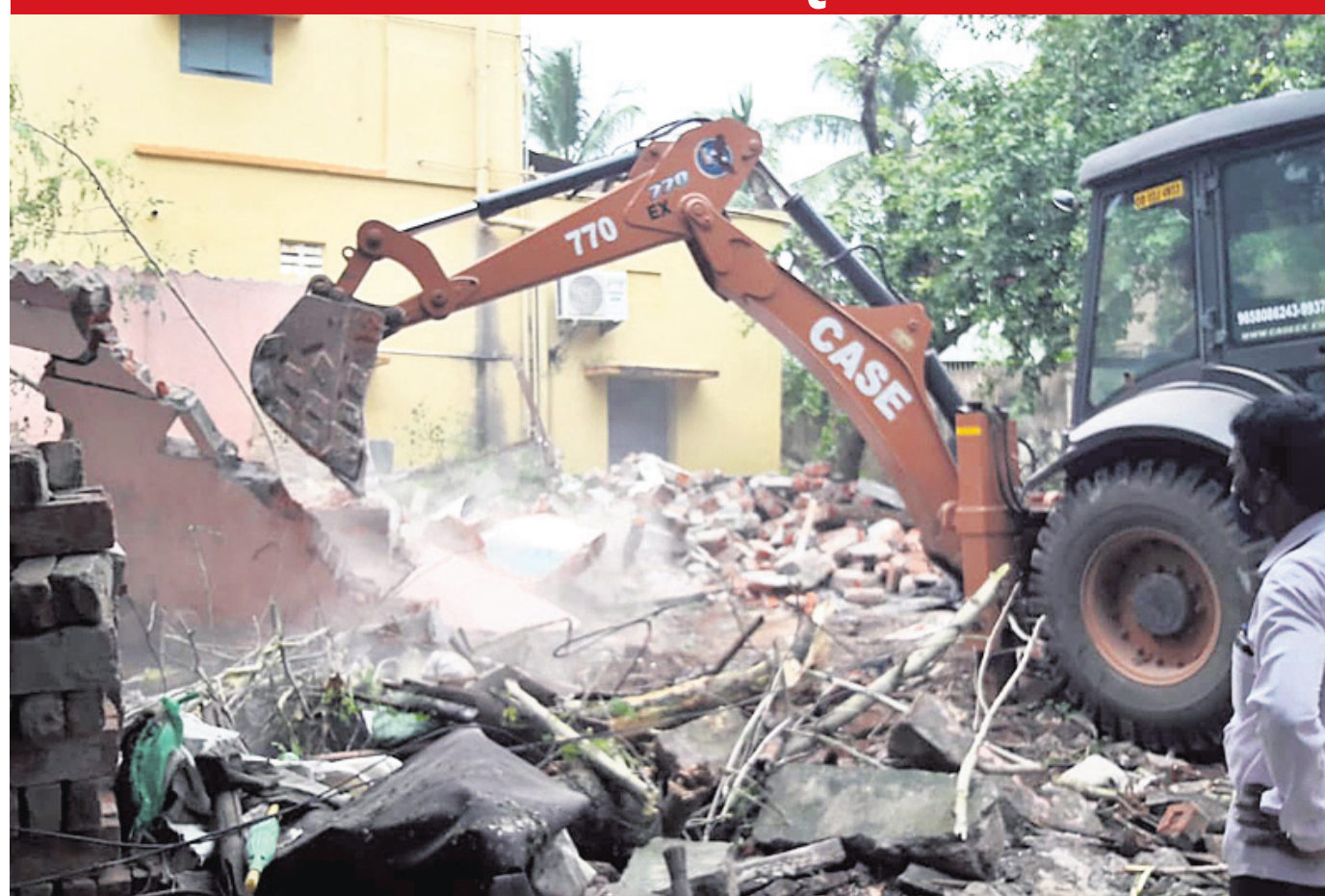
Civic authorities in Bhubaneswar demolish illegal structures at Sahid Nagar, Tuesday
