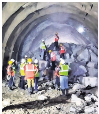
Completion of the Railway proj-
