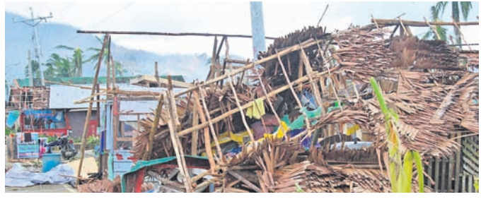
A house damaged by Typhoon Rai lies along a road in Surigao del Norte province, southern Philippines
