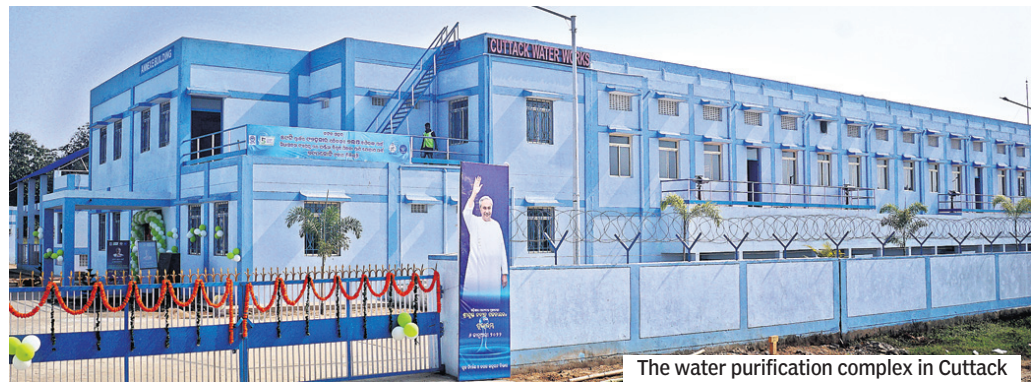
The water purification complex in Cuttack
