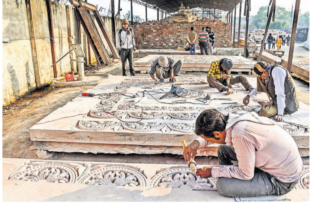
A worker carves stone as part of construction of Ram Temple in Ayodhya, Sunday.
