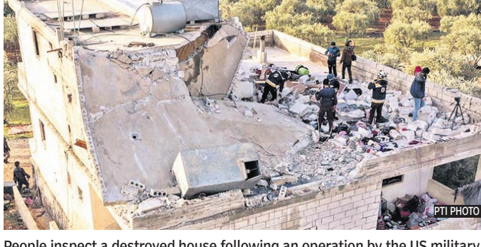
People inspect a destroyed house following an operation by the US military
