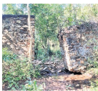
bridge across Ramial river to reach Hati-Girida.
