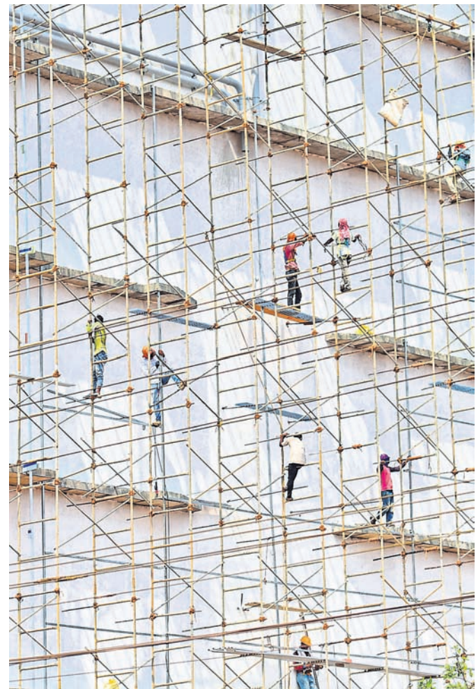
TOILING HARD: labourers work on an under-construction building in udupi, karnataka
