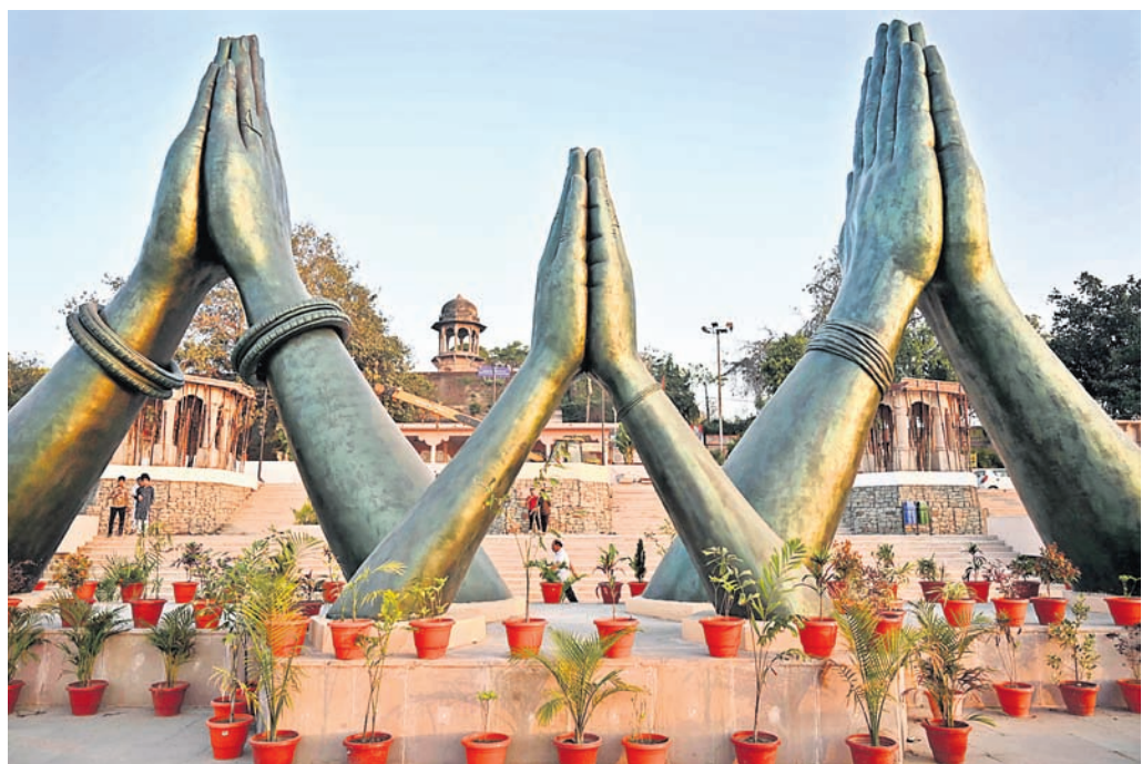
A view of Khidkiya Ghat on the banks of River Ganga in Varanasi during the renovation work Sunday. The ghat is named so because it is like a window to Varanasi from where the crescent shape of the Ganga flowing is clearly visible. PTI PHOTO
