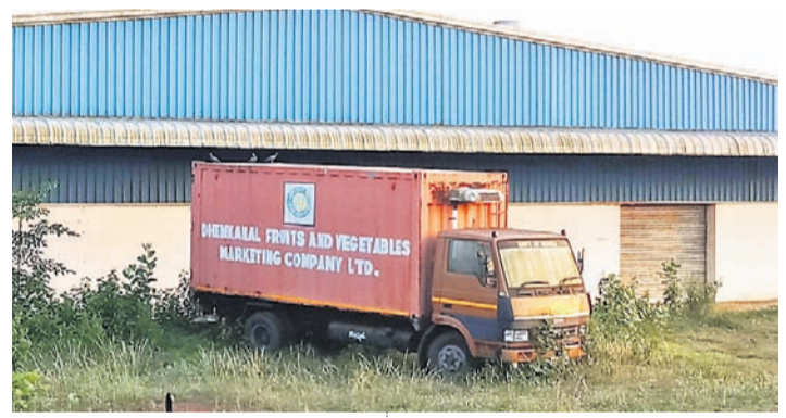
HORTICULTURE BOOST Chief Minister Naveen Patnaik had laid the foundation stone for the hub June 27, 2013 at Gobindpur near NH-55 under Sadar block in the district
