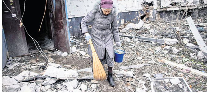
A woman holds a broom outside a heavily damaged apartment block, following an artillery attack in Ukraine REUTERS PHOTO
