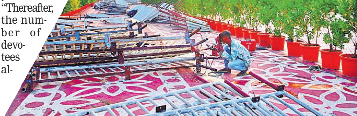
Re-barricading work in progress near Srimandir, Saturday
