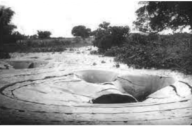
Liquefaction during the earthquake
