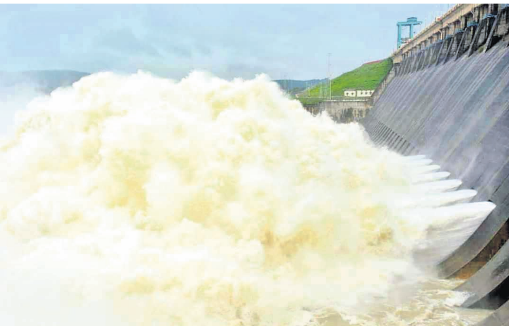
Five sluice gates of the Hirakud dam were opened Thursday as the water level rose to 605 feet against the optimum level of 630 feet due to incessant rains in Sambalpur district
