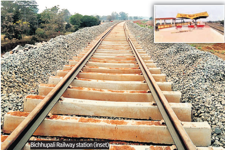
Bichhupali Railway station (inset)
