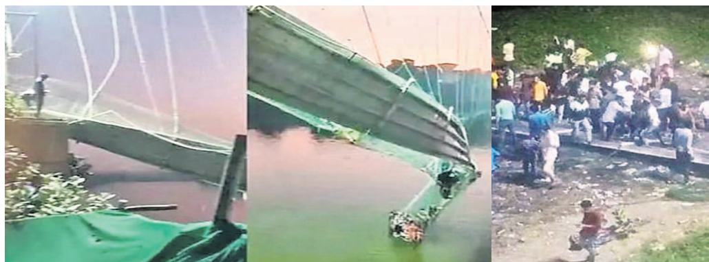
The suspension bridge, which reopened just 4 days back after 7 months of repair work, had not received any 'fitness certificate'
