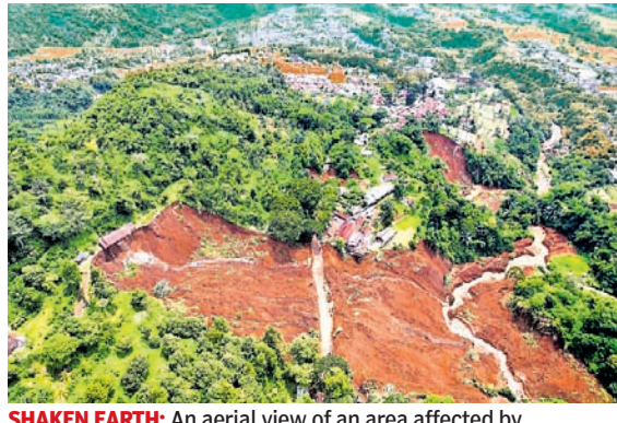
SHAKEN EARTH: An aerial view of an area affected by landslides following earthquake in Cianjur
