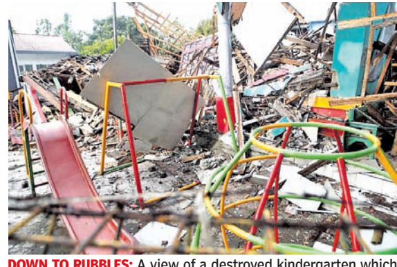
DOWN TO RUBBLES: A view of a destroyed kindergarten which was affected by the earthquake in Cugenang
