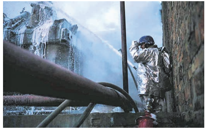
A firefighter works at a site of a critical power infrastructure object which was hit during Russia's drone attacks in Kyiv
