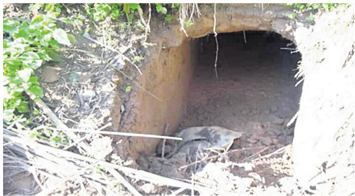
The BSF has unearthed at least five under-ground tunnels in the about 192 km of the Jammu front (of the India-Pakistan IB) in the last three years
