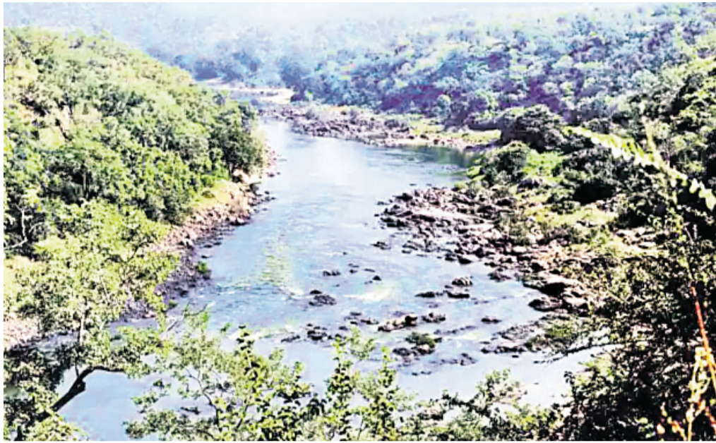
puted Kalasa-Bhanduri dam.
